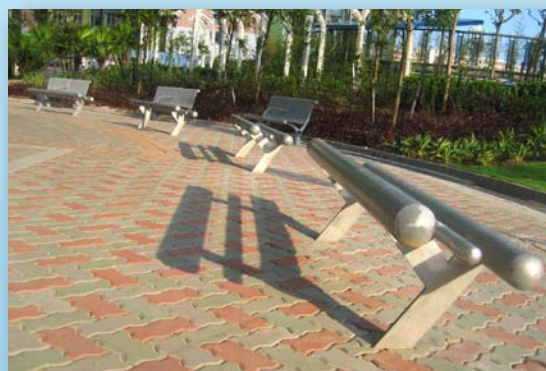
以回收玻璃物料製成的環保地磚鋪設而成的行人路。 Pedestrian walkways paved by eco-bricks made with recycled glass aggregates.
